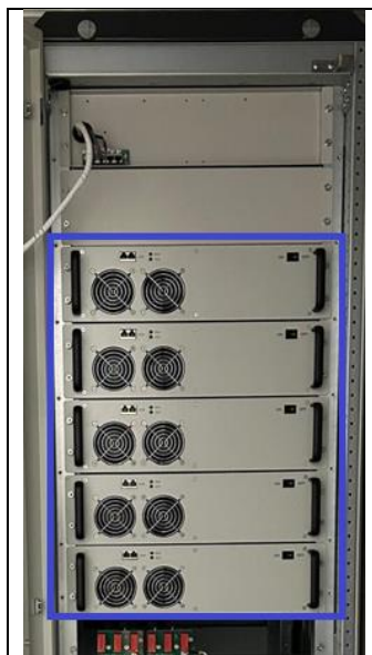
Figure 7: HPS250 Split Unit MPPT Slots Example
